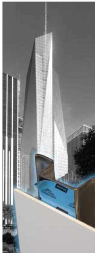
NORMOUNT V2800H on Architectural Panels — Bank of America Tower (New York City)
